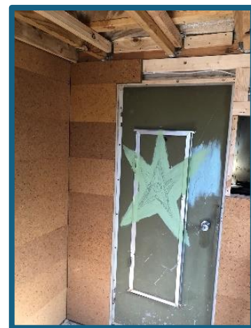
Cladding around the door in the cork
