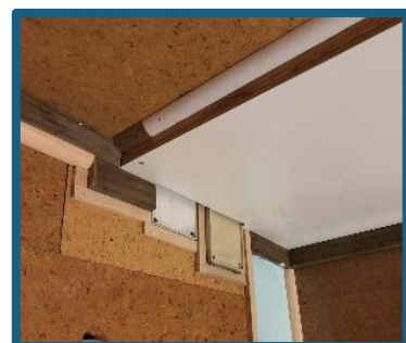
The thin pine board around tight spaces
