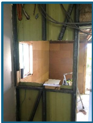
After cutting the holes
