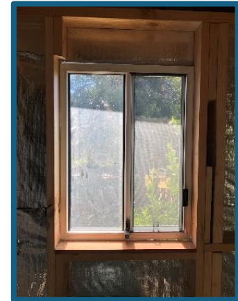
The window installed
