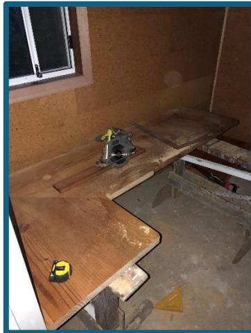
Me cutting the desk down to size, as well as the 45-degree corner off late at night
