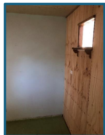
The Live room clad in ply and the new window framed
