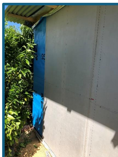
Putting up the cement board
