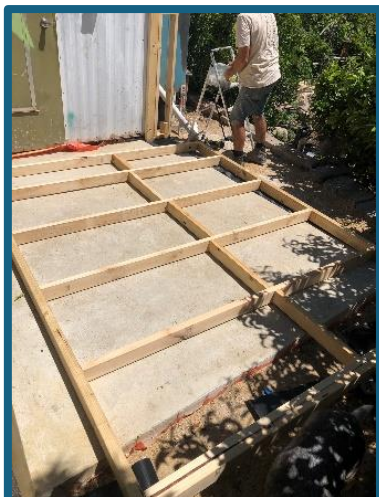
Building the frames flat on the slab
