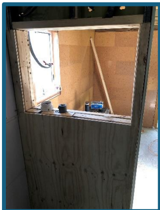
After framing and cladding
