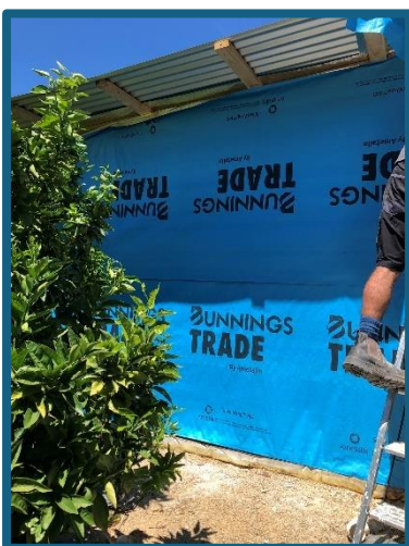
Wrapping the frame in silver wrap
