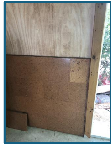
Cladding the walls in the cork
