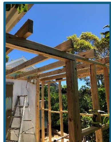
The frame finished
