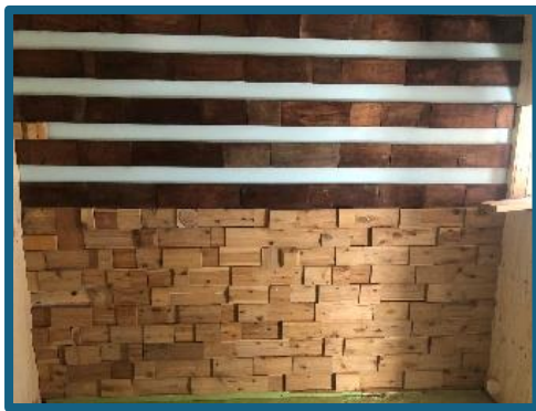
The wall complete
