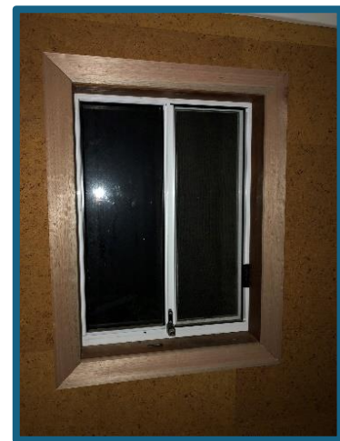
The trim around the window in the control room
