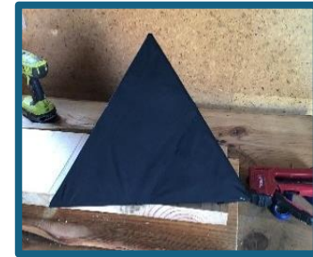
Covering In fabric and filling with insulation
