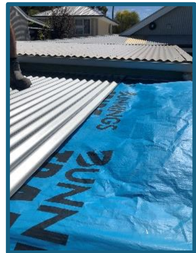
A photo showing the building of the roof
