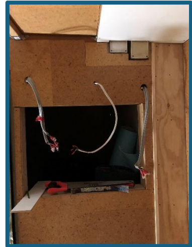
Running the wires through the cladding
