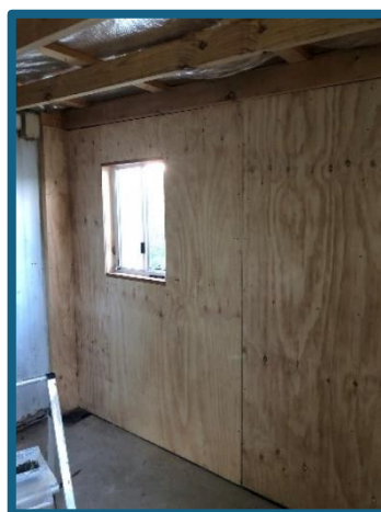
The control room clad in ply
