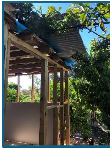
The finished roof, showing the cramped space we worked in
