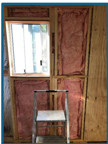
Insulating and cladding around the window in the control room
