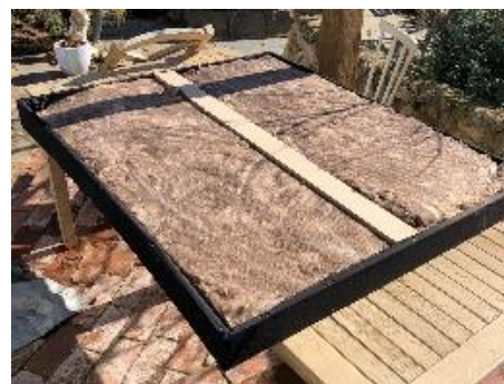
Me stretching and stapling the material, then adding insulation
