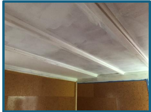
Painting the control room ceiling
